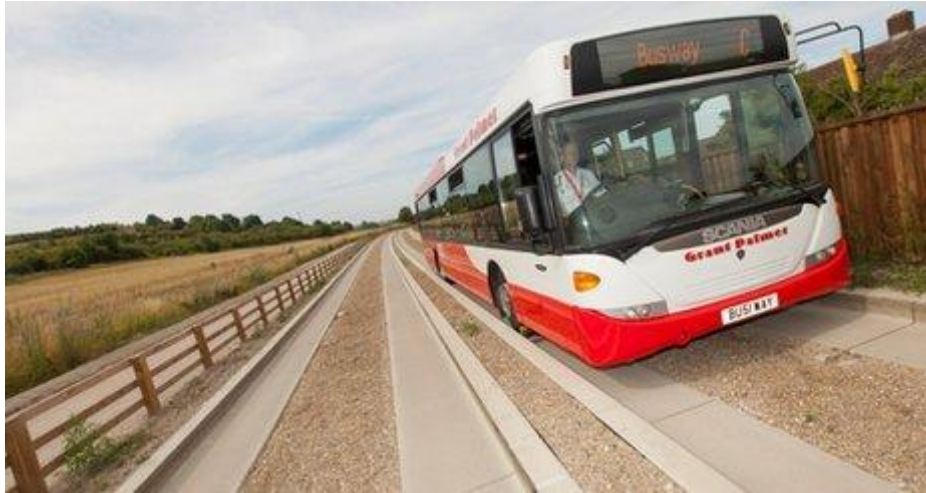
Figure 6: Luton-Dunstable Busway (courtesy of Luton Borough Council)
